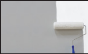
Cat Basecoat Decorshield 2x lapis (by roll)
