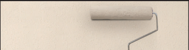
Cat Akhir Interior : Decorcryl/Decorlotus Exterior : Decorshield/Decorflex 2x lapis (by roll)
