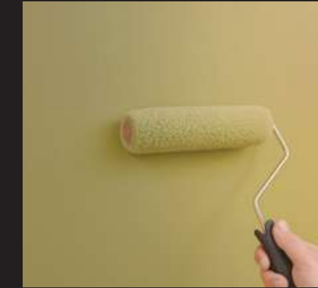
Cat Basecoat Decorshield (tinting color) 2x lapis (by roll)
