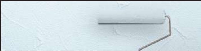
Cat Akhir Interior : Decorcryl/Decorlotus Exterior: Decorshield/Decorflex 2x lapis (by roll)
