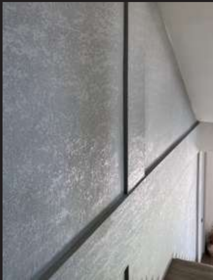
DTX -250 | Villa Ungasan, Bali
